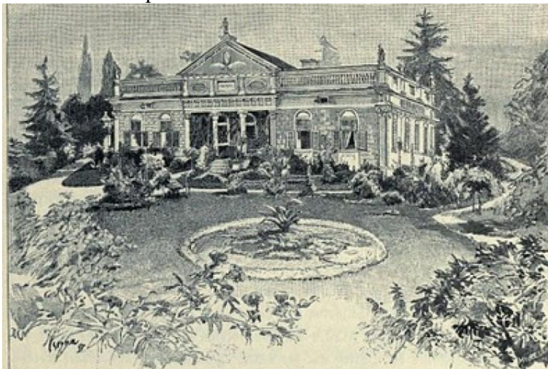
Figure 2. The original image of the Berhlen castle, from Chiraleș (Source: http://www.monumenteuitate.org/ro/monument/56/Chirales-Bethlen )
